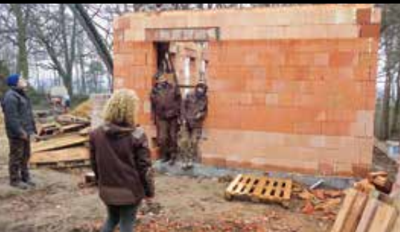
Stavba provozovny gastru /The construction of the restaurant establishment/
