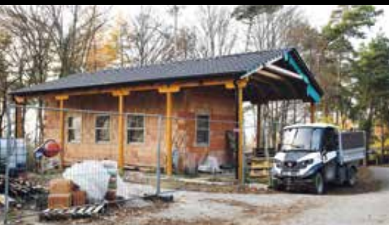
Stavba provozovny v listopadu 2021 /The construction of the establishment in November 2021/
